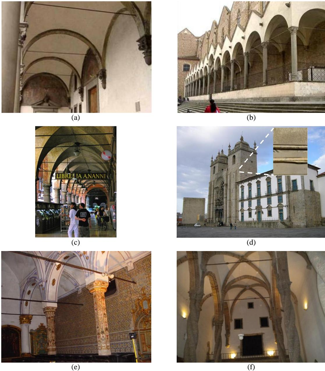
Figure 5.24 – Examples of tie-rods in existent masonry structures: (a) circular bars in the Ospedale degli Innocenti, Florence, Italy; (b) circular bars in the Santa Croce, Florence, Italy; (c) rectangular bars in the via Zamboni, Bologna, Italy; (d) circular bars in the cathedral of Porto, Portugal; (e) and (f) rectangular bars in the Jesus' Church, Setúbal, Portugal
