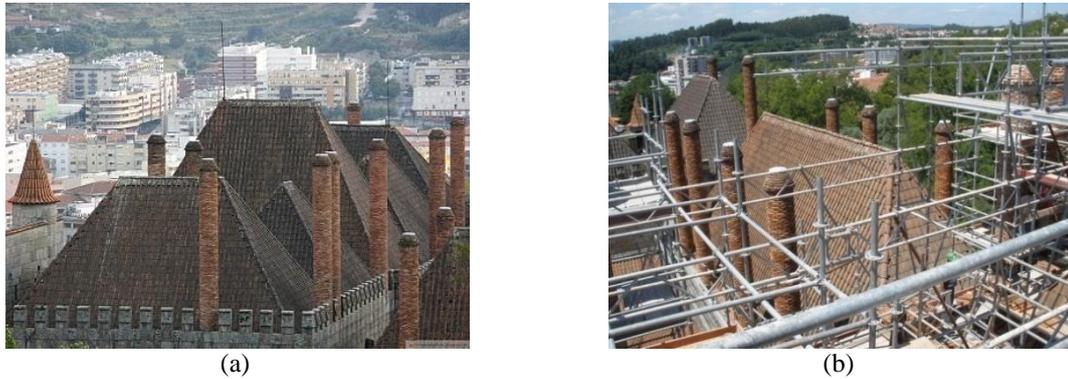
Figure 4.25 – Chimneys at Paço dos Duques building: (a) general view; and (b) conservation works
